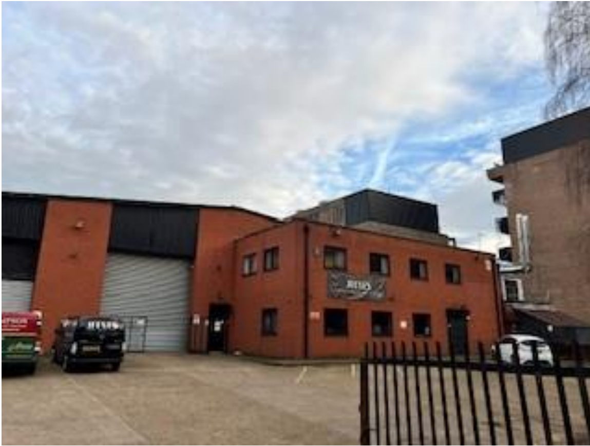
Site photos – Existing Commercial Unit (laundry)
