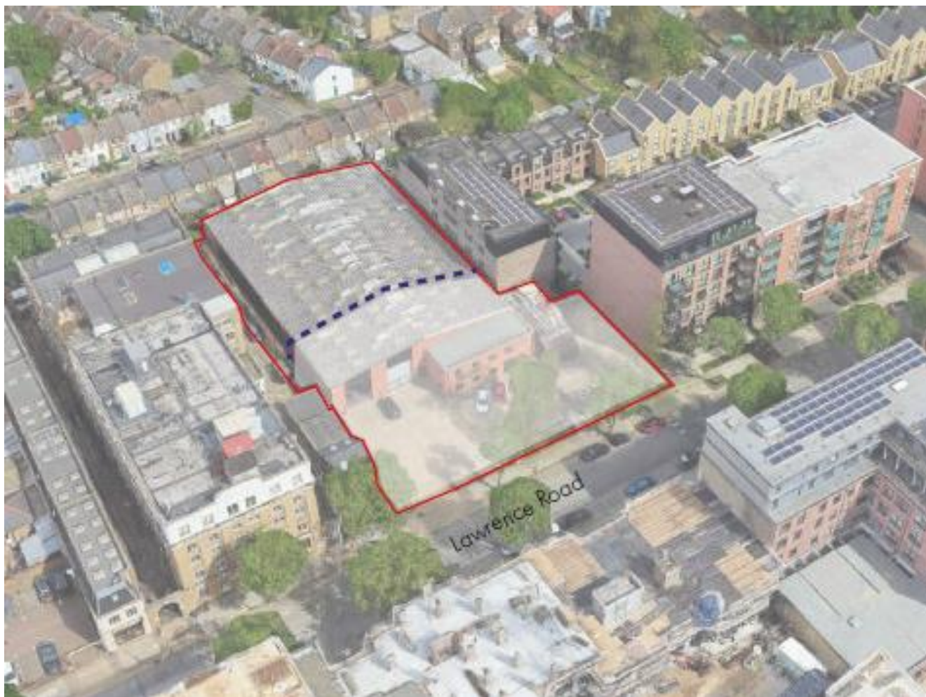
Fig 1: site location in context
